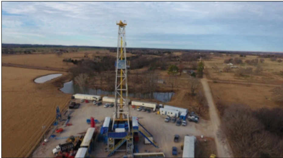
BNK Drilling Rig #2
